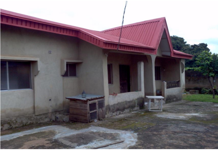
Figure 5 A semi-detached twin bungalows at Akobo, Ibadan
