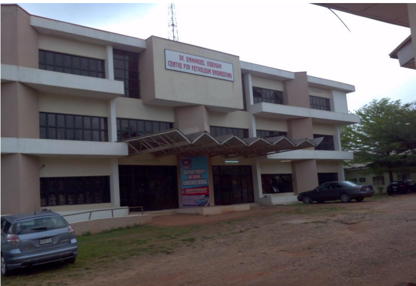
Figure 6 Dr Egbogah's building (Department of Civil Engineering, University of Ibadan)
